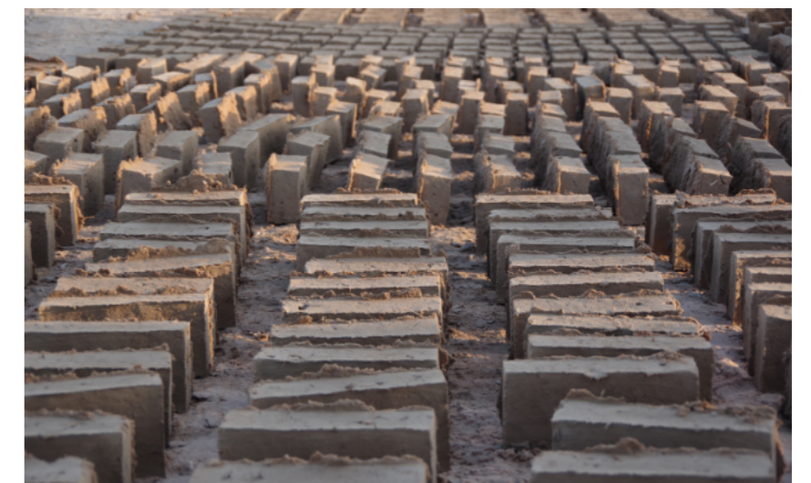
Earth block production on site under supervision of SBAH © J. A. Blaschek (ZRSI)
