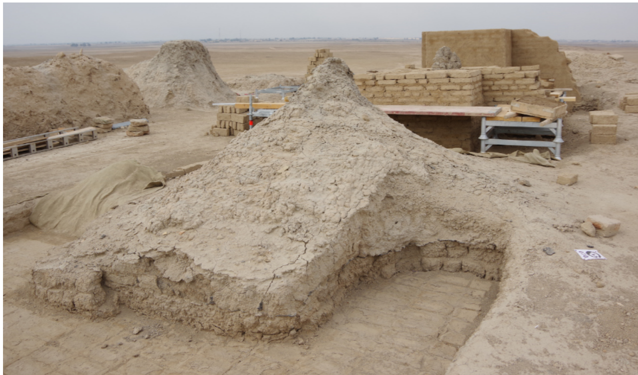
Completion of the soil consolidation (left) | emergency securing supplementation of the original finding (centre) | completion of the supplementation work (back). © J. A. Blaschek (ZRSI)
